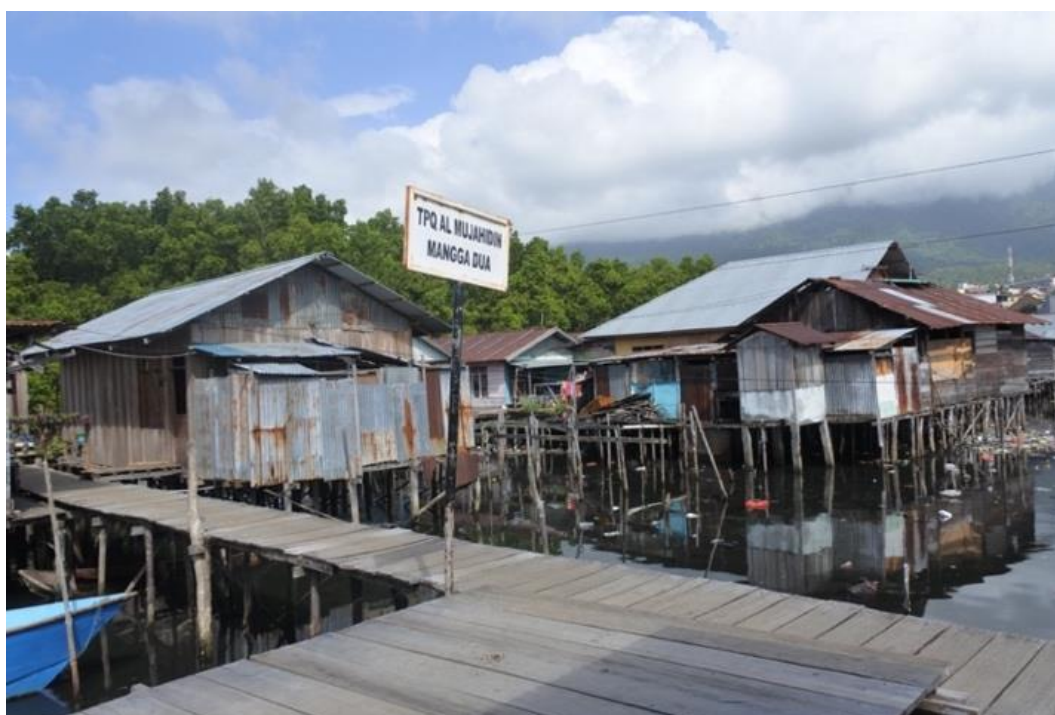
Figure 10. Environment conditions in Mangga Dua Utara District.
