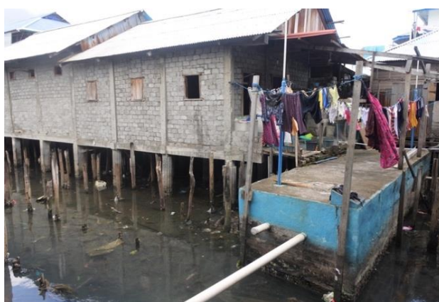
Figure 4. Conditions of the drainage channel.
