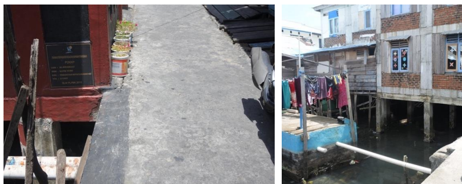
Figure 6. Communal septic tank.
