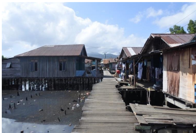
Figure 11. Conditions were existing of sewerage.
