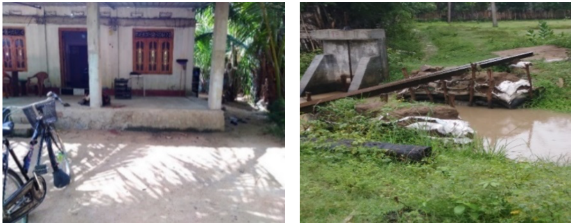
Figure 4. Left: Foundation of a house, Right: Temporary small bridge (source: field study, 2019).
