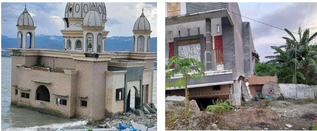
Figure 1. (a). The tsunami damaged the mosque; (b) Houses sank into the ground due to liquefaction. Documentation by Team
