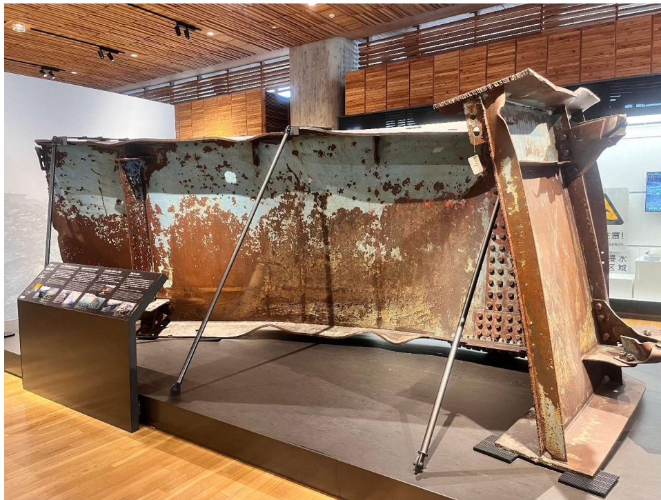
Figure 2. Kesen Ohashi Bridge Part Damaged by Tsunami Disaster, Source: Author (2024).
