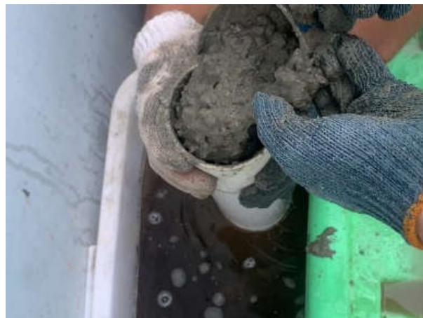
Gambar 1. Pengecoran Underwater Concrete
